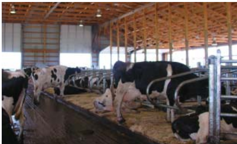
The building area of the free-stall barn is 1,967 m 2 (21,176 ft 2 ). Designed by Curry-Wille and Associates, it is the first working agricultural building to seek Leadership in Energy and Environmental Design, or LEED, certification. Among other energy efficient and resource conservation features, the barn uses an automatic sidewall curtain system that raises or lowers to regulate temperature, which maximizes sunlight and reduces the need for electric lighting. (Photos by Laing and Mitrovich)
